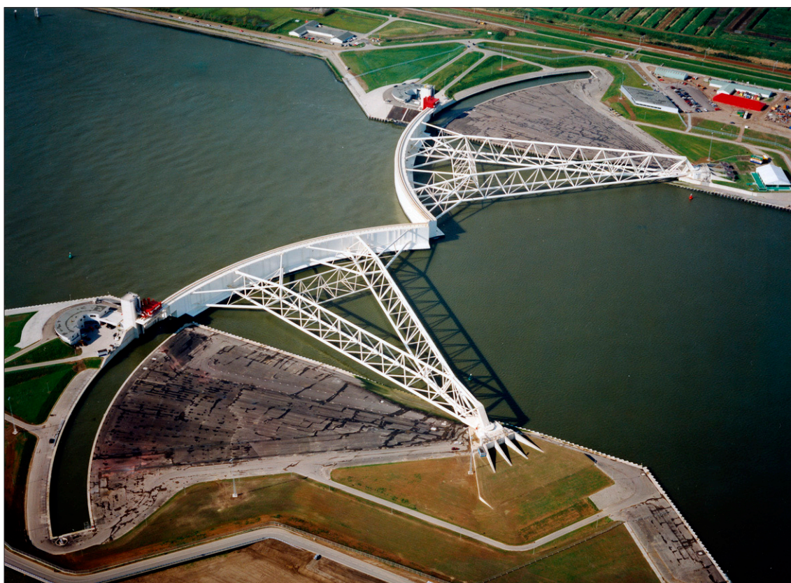
Figure 5. The Maeslant storm surge barrier near Rotterdam during a test closure (source: www.BeeldbankVenW.nl ).
